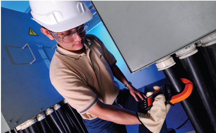
Figure 2. Large jaw clamp opening of 52mm / 2 inches
