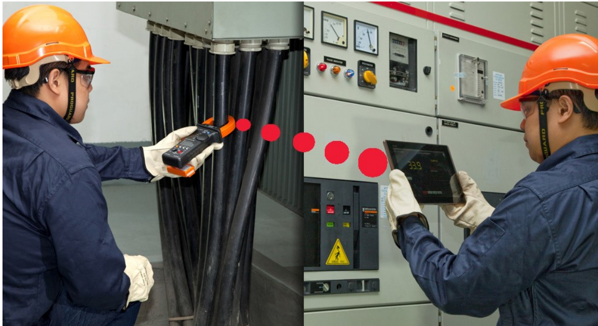
Figure 4. Monitor measurements and log data up to 10-meters range across all Android platform devices with the U1177A Infrared-to- Bluetooth adapter.
